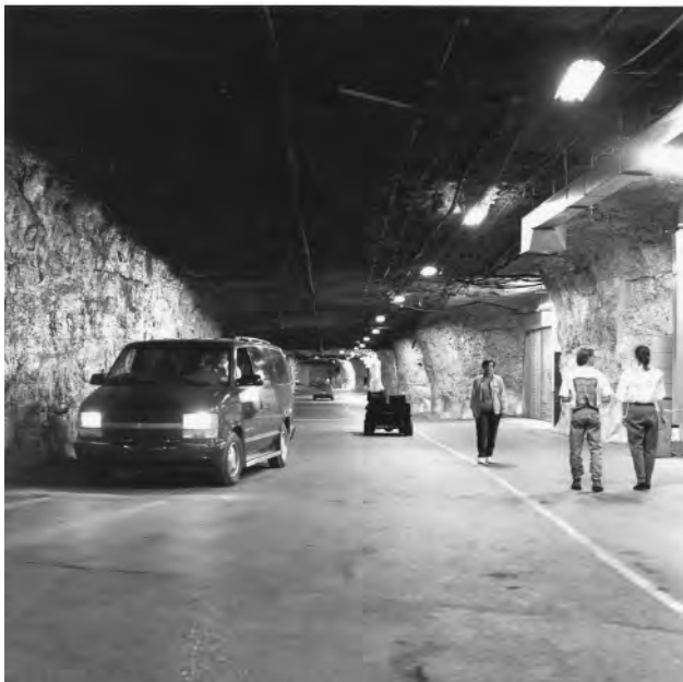
Fig. 9 (a) Entering the Iron Mountain underground storage facility. (b) Inside the roadway of Iron Mountain. (Courtesy of National Underground Storage, Iron Mountain, 2001.)
