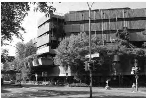
Fig. 14 Freiburg University Library, a typical building of the late 1970s. (Source: Freiburg University Library.) (View this art in color at www.dekker.com .)
