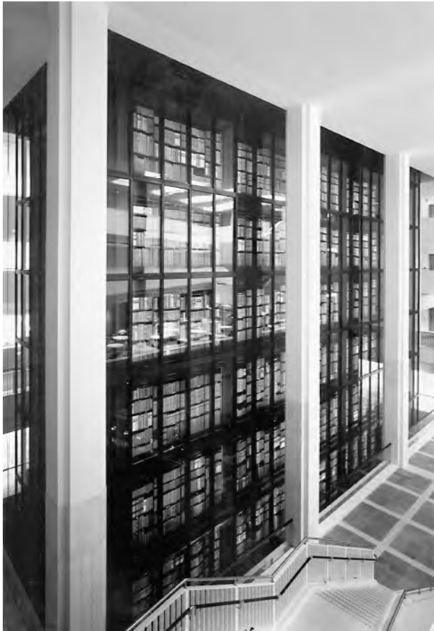
Fig. 6 The tower of the King's Library, St. Pancras. ( Go to www.dekker.com to view this figure in color. )
