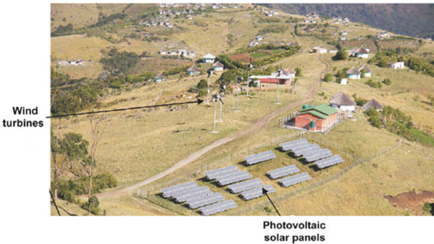
Fig. 51 The Lucingweni Village mini-hybrid off-grid system
