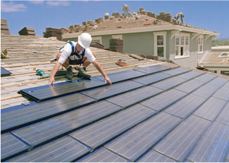
Fig. 3 Qualified person in maintenance activities
