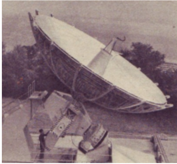
Fig. 1 Solar oven, diameter 50 m, 3,000 °C (Algiers)
