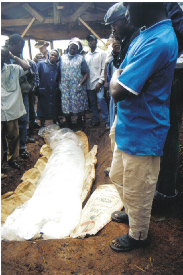
Fig. 12 The completed digester in Cameroon
