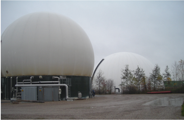
Fig. 6 Manure storage tank ( front ) and gas storage facility at Hashøj biogas plant ( Photo by author, [47])
