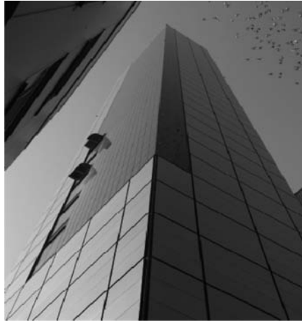
Figure 3.9 Grain silo 'Schapfenmühle' on the outskirts of Ulm, Germany. 1306 CIS modules from the Würth Solar pilot plant with a nominal installed power of 98 kWp are integrated into the façade (Source: Powalla & Bennet 2007, Hindawi Publishing Corp., Copyright © 2007 M. Powalla & D. Bonnet)
