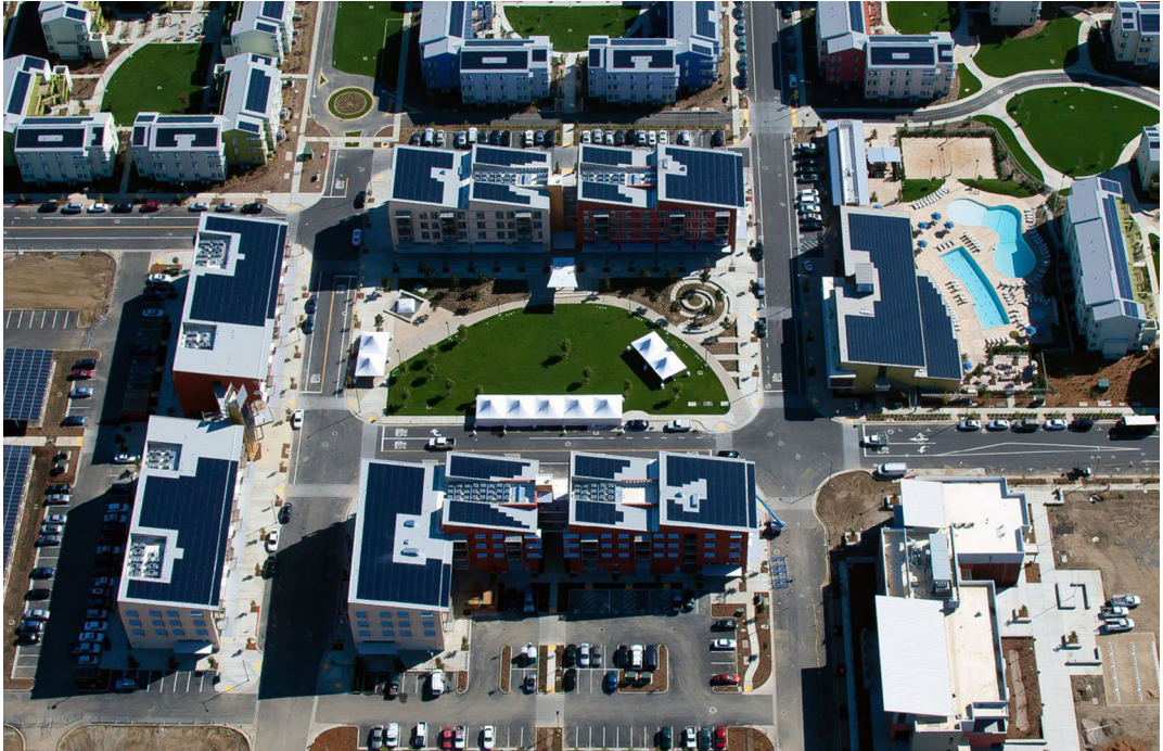
FIGURE 20.2 Aerial view of 4.1 MW of integrated solar energy at the UC Davis West Village. West Village is the largest net zero energy community in the United States, combining energy efficient technology with on-site energy production via rooftop and vertical photovoltaic installations (Davis, California). Photo courtesy of UC Davis.
