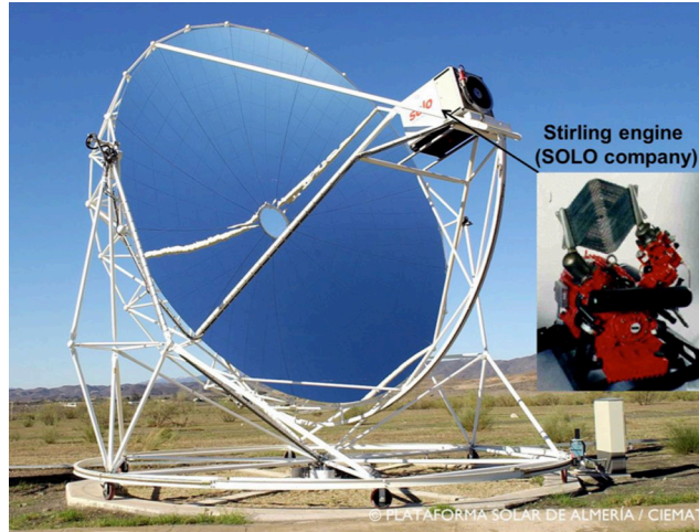
FIGURE 7.10 One of the parabolic dishes installed at the Plataforma Solar de Almería ( www.psa.es ).
