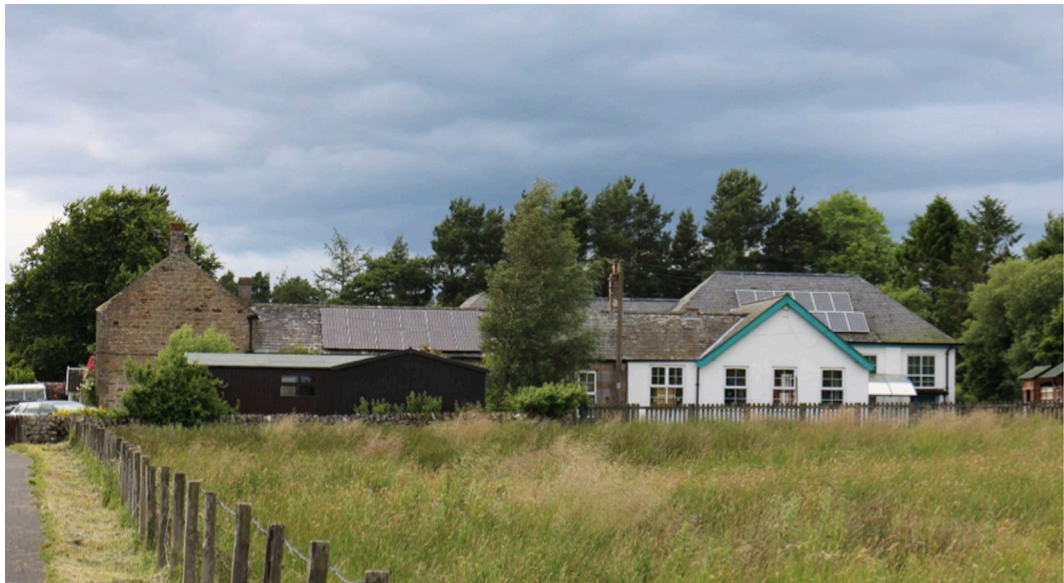
FIGURE 19.2 Solar panels retrofitted onto existing buildings, Otterburn First School, Northumberland UK. Photo: B. Dower (all rights reserved).
