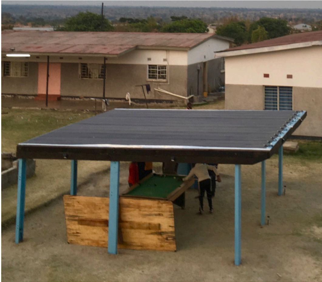
FIGURE 5.2 Photograph of build in Mutende, Lulamba, Zambia with twelve 136 W amorphous Si PV panels with an inverter/charger for two 102 Ah lead acid batteries feeding a mains outlet. A small DC system powers internal lighting (six LED bulbs) a radio and two USB charging points through a small battery bank.
