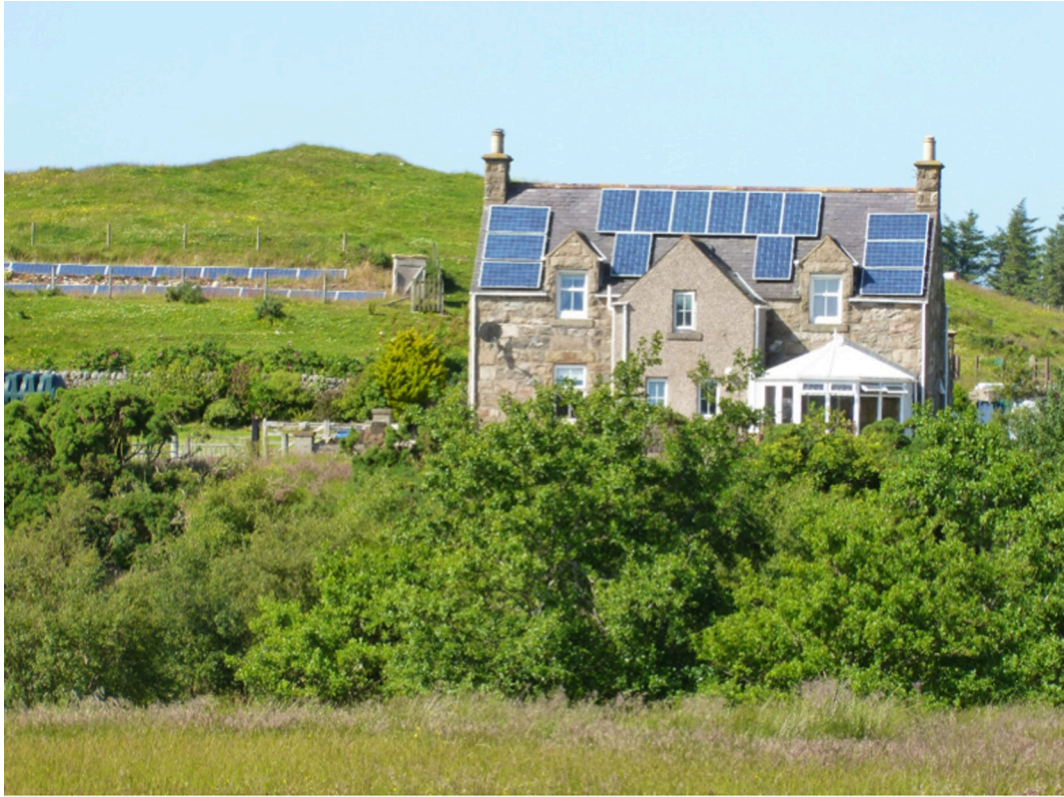
FIGURE 19.4 Solar panels ruin the appearance of this vernacular style house in northern Scotland. The better sited panels are those in the garden behind. Photo: B. Dower (all rights reserved).
