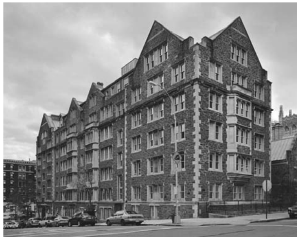
Figure 6.11 Knox Hall of Columbia University. Knox Hall of Columbia University, a century-old historical building, is located at 606 West 122nd Street, Manhattan. During a 16-month-long renovation, ended on February 2010, one of the largest shallow geothermal energy facilities in New York City was installed. It has four 1800-ft (547 m) geothermal wells and heat pumps for both heating and cooling. The only visible marks of the project on the exterior of this historical building are four covered manholes on the sidewalk. Courtesy of Columbia University.
