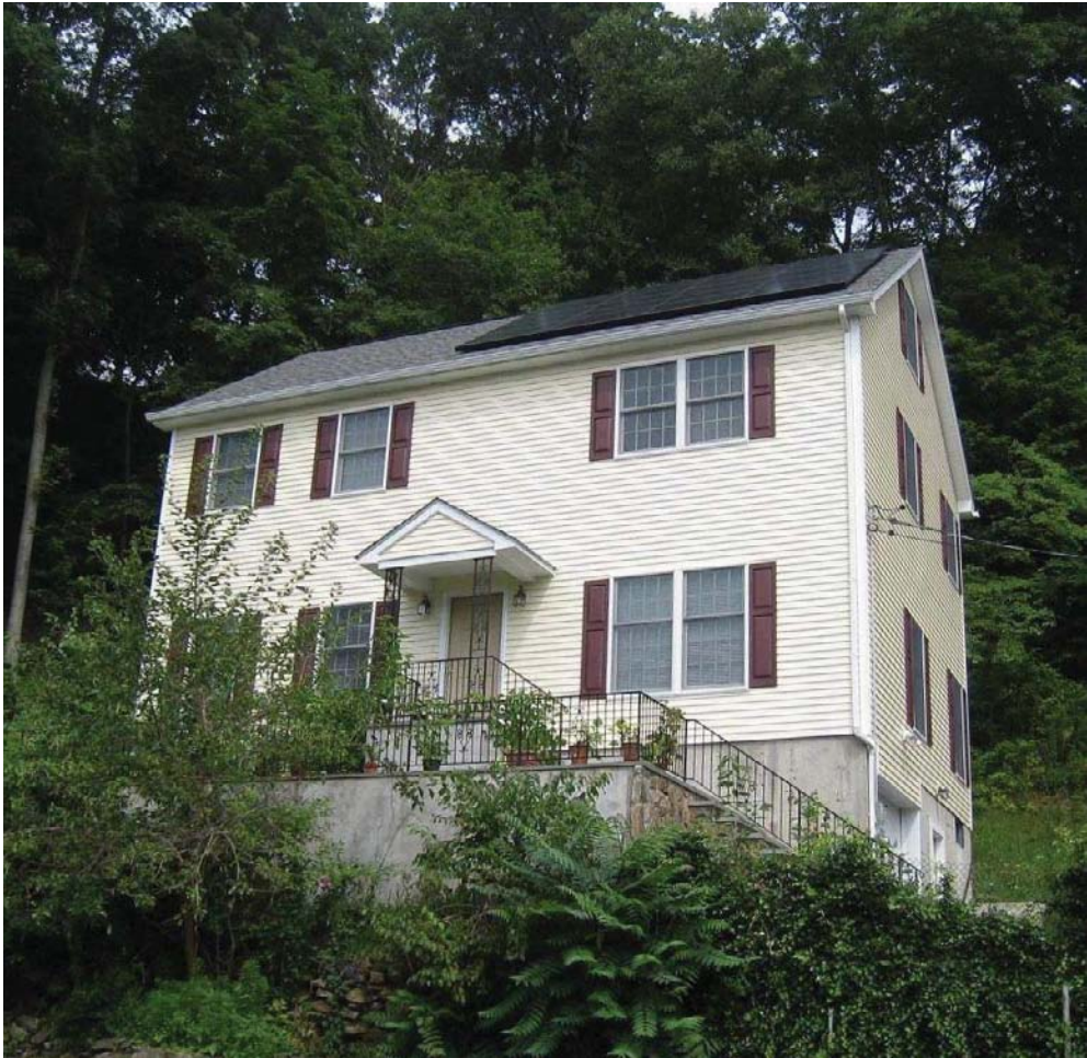
Plate 16. An experimental solar house. As Steven Chu repeatedly advocated, using better building design to take advantage of solar energy, with a small incremental investment, tremendous energy savings can be achieved. Shown here is an experimental single-family house designed by the author. It is a medium-size central-hall colonial house very common in the United States. Nevertheless, the layout, roof design, and window placement are optimized for solar energy utilization. On a sunny winter day, the sunlight through the large south-facing windows warm all the often-occupied rooms such that the thermostat for gas heating is always turned off. In the Summer, the solar panels on the roof drive two central air-conditioning systems to keep the entire house cool. A solar-powered attic fan (on top of the roof, not shown here) further reduces the cooling load. The walls are well insulated and all windows are double pane, air tight, and filled with argon. See Section 13.3. Photo taken by the author.
