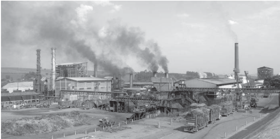
Figure 1.13 Costa Pinto Production Plant of sugar ethanol. The foreground shows the receiving operation of the sugarcane harvest; on the right in the background is the distillation facility where ethanol is produced. Courtesy of Mariordo.
