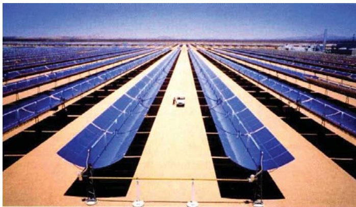
Plate 11. Parabolic trough concentrators at Kramer Junction, CA. The system, called the Solar Electricity Generating System (SEGS) installed at Kramer Junction in Mojave desert, California, starting from 1984. The SEGS system is the largest solar electricity generator set on the world. The total capacity is 354 MW. See Section 11.4.
