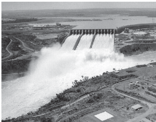
Figure 1.9 Itaipu hydropower station at border of Brazil and Paraguay. With a capacity of 14.0 GW, the Itaipu hydropower station is one of the world's largest and generates about 20% of Brazil's electricity.
