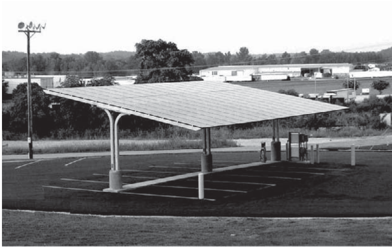
Figure 12.11 Solar-powered electric car charging station in Tennessee. In the United States, taking another step in building its electric vehicle charging infrastructure, Tennessee is now home to the first of several solar-powered EV-charging stations [10].
