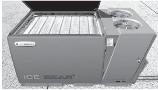
Figure 12.3 Ice Bear energy storage system. An insulated tank is filled with water and many copper heat exchange coils. During the night, the refrigerator uses inexpensive electricity and cool air to make ice from the water. As shown in Chapter 6, the lower the ambient temperature, the higher COP. Therefore, to make a well-defined mass of ice during the night, the electricity cost is much lower than in the hot daytime. Courtesy of Ice Energy, Inc.
