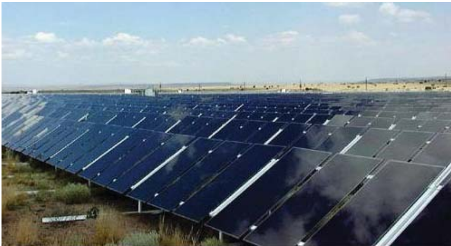
Plate 7. Utility-scale CIGS thin-film solar field. Thin film solar cells use much thinner semiconductor materials than crystalline solar cells, thus the cost per watt could be much lower. See Section 9.6. Shown here is a 750 KW CIGS solar panel system installed in Tucson, AZ, manufactured by Nanosolar. Photo courtesy of Nanostar Inc.
