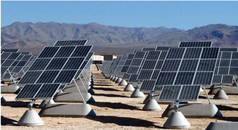
Plate 6. Crystalline silicon solar cells with single-axis tracking. The Nellis Solar Power Plant, located within Nellis Air Force Base in Clark County, Nevada, with a peak power generation capacity of approximately 14 MW. A simple uniaxial sunlight tracking system can increase the power output by 60% from the optimum fixed-orientation system, see Section 4.3.4. Photo courtesy of U.S. Airforce.
