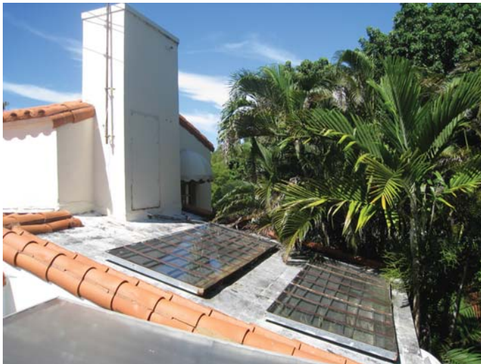
Plate 14. Day-and-Night solar water heaters manufactured and installed in 1920s in Maimi. Solar water heaters (see Sections 1.5.1, 11.2, and 11.3) can be very durable. In the 1920s, about 40,000 Day-and-Night solar water heaters were installed in Florida. After 80 years of operation in violent weather conditions, thousands of them are still working properly today. The secret is its simplicity and complete absence of moving parts. Photos taken by the author, August 2010, Miami.
