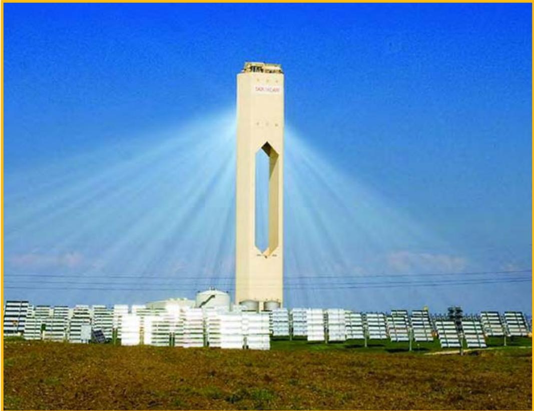
A solar power tower is another solar thermal power plant design. Thousands of flat, moveable mirrors called heliostats surround a tower. The heliostats direct sunlight to the top of the tower where tubes filled with liquid sodium collect the solar heat. Liquid sodium gets very hot, at least 1200 degrees Fahrenheit (649 degrees Celsius). The salty liquid holds heat better than water or oil. The heat produces steam for electricity, or it is stored and used later when there is no sunshine.
