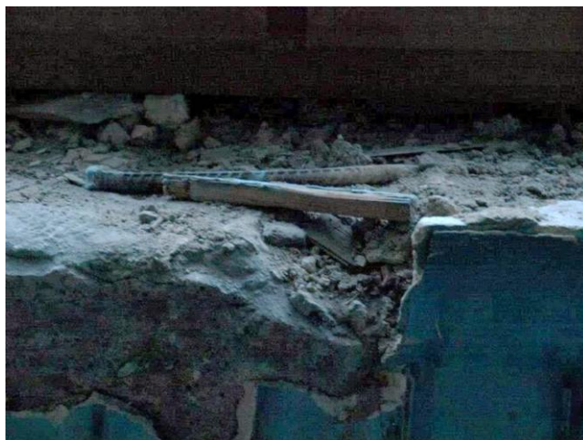
Window frame inside of a home in Telavi center after rehabilitation of building façade. Photo by Tinatin Zurabishvili
