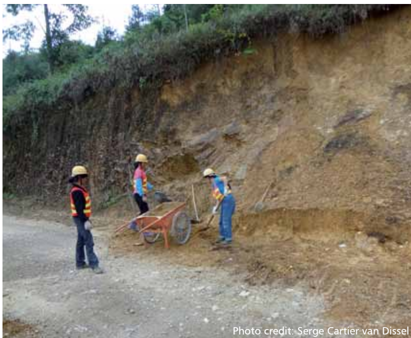
Yunmao group removing a landslide
