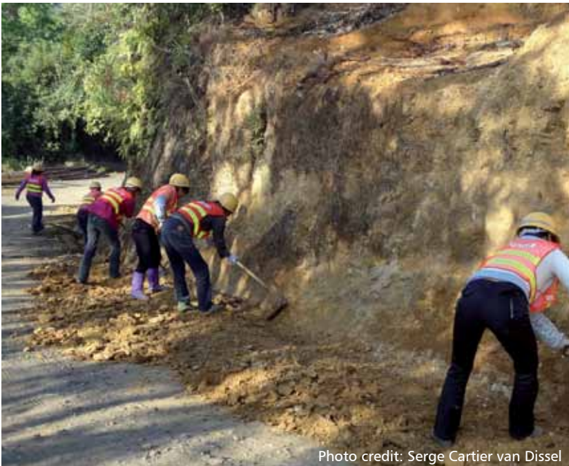
Hexinchang group creating a side drain
