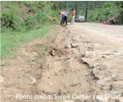
Road shoulder in poor condition
