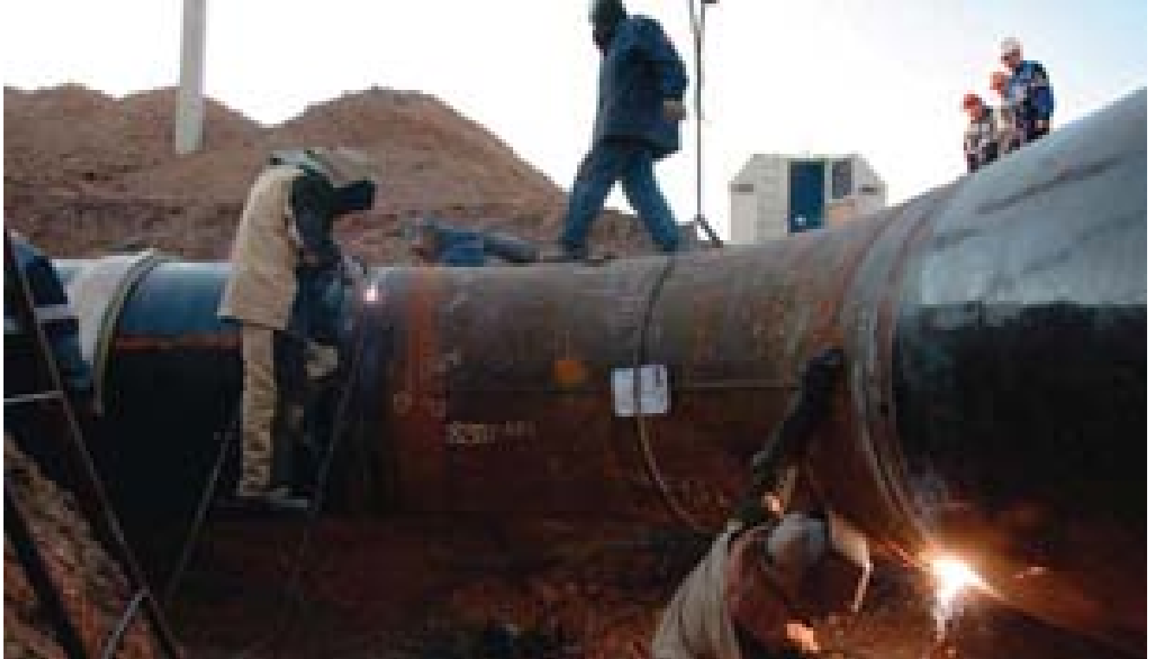
■ Gazprom welders work on a pipe during reconstruction works on the pipeline in Alexandrov Gai village at the border between Kazakhstan and the Russian Federation. The pipeline is expected to increase the possibilities of gas transport from Central Asia to Europe.
